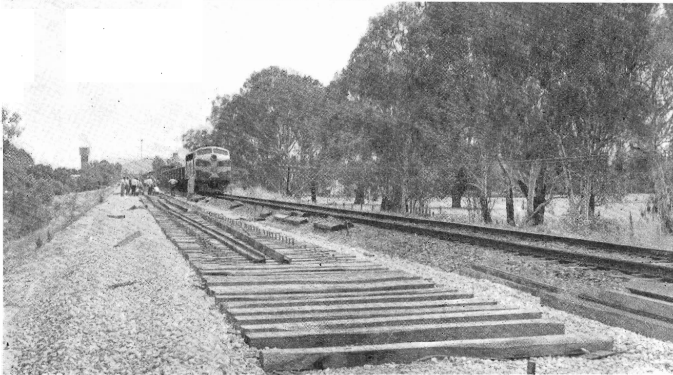
STANDARD GAUGE TRACK LAYING
